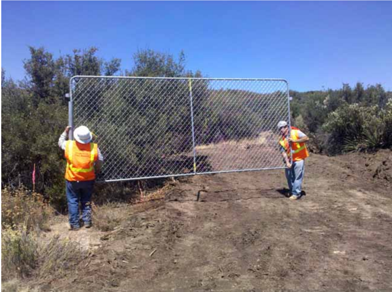
Temporary fence installation at EP126. Photo courtesy of Rosina Gallego.
